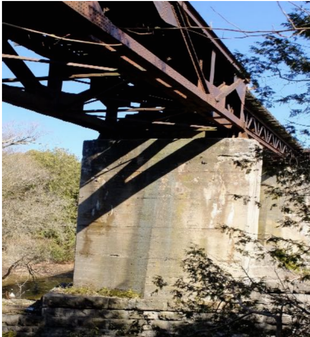
Trestle Bridge stone pier
